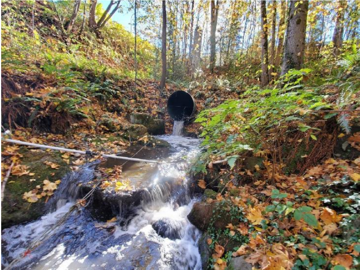
Figure 2C - Existing Culvert Outlet
